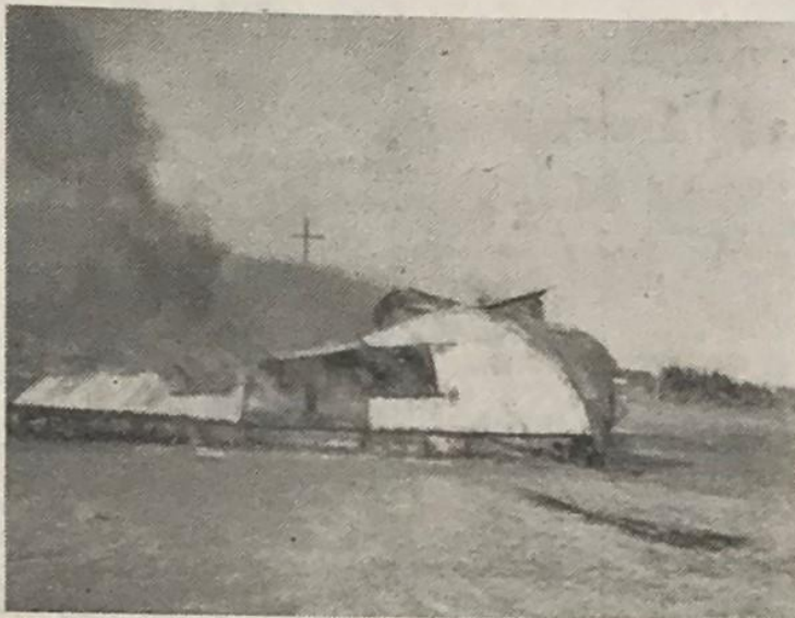
Above is a view of the Church at Deer Park being destroyed by fire.
